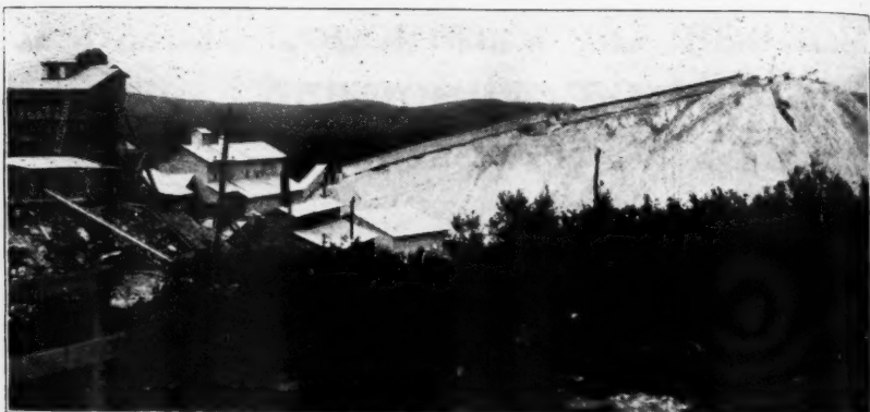
Left to Right, Secondary Crusher and Dryer; the Mill Tailings Belt Conveyor
